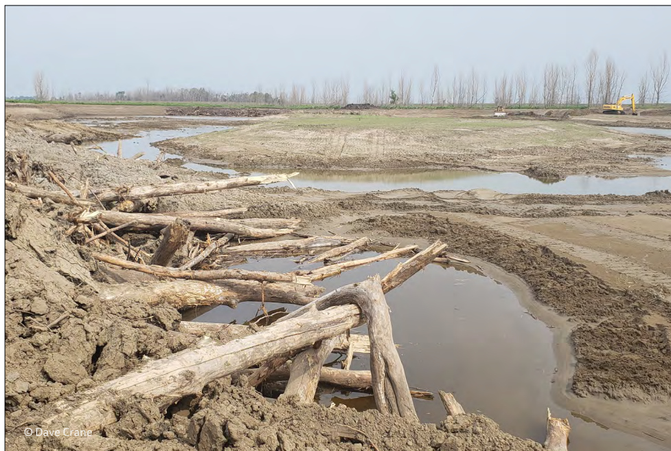
Large woody debris placement and fine grading at borrow pit wetland site.
