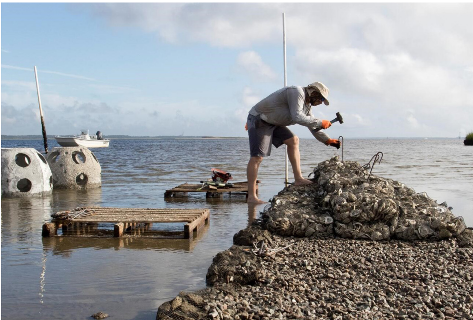
Building an oyster reef with bagged oyster shells and reef balls at Shellbed Island in the Lower Cape Fear River, North Carolina.
